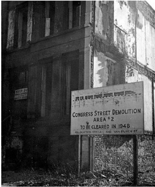
Figure 15 In the bulldozers path
