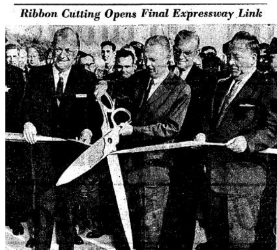
Figure 17 The Highway is Open! - October 12, 1960
