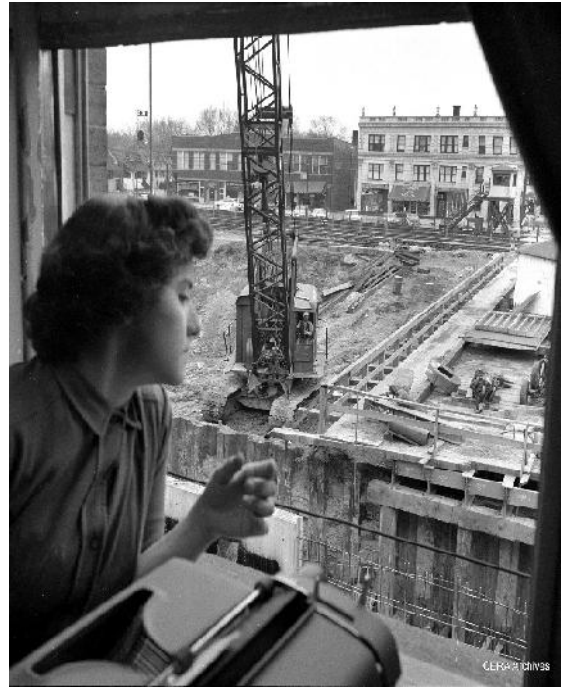
Figure 16 Digging the Oak Park trench
